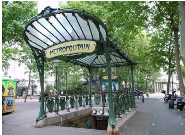
High quality Metro station entrance Paris, France
