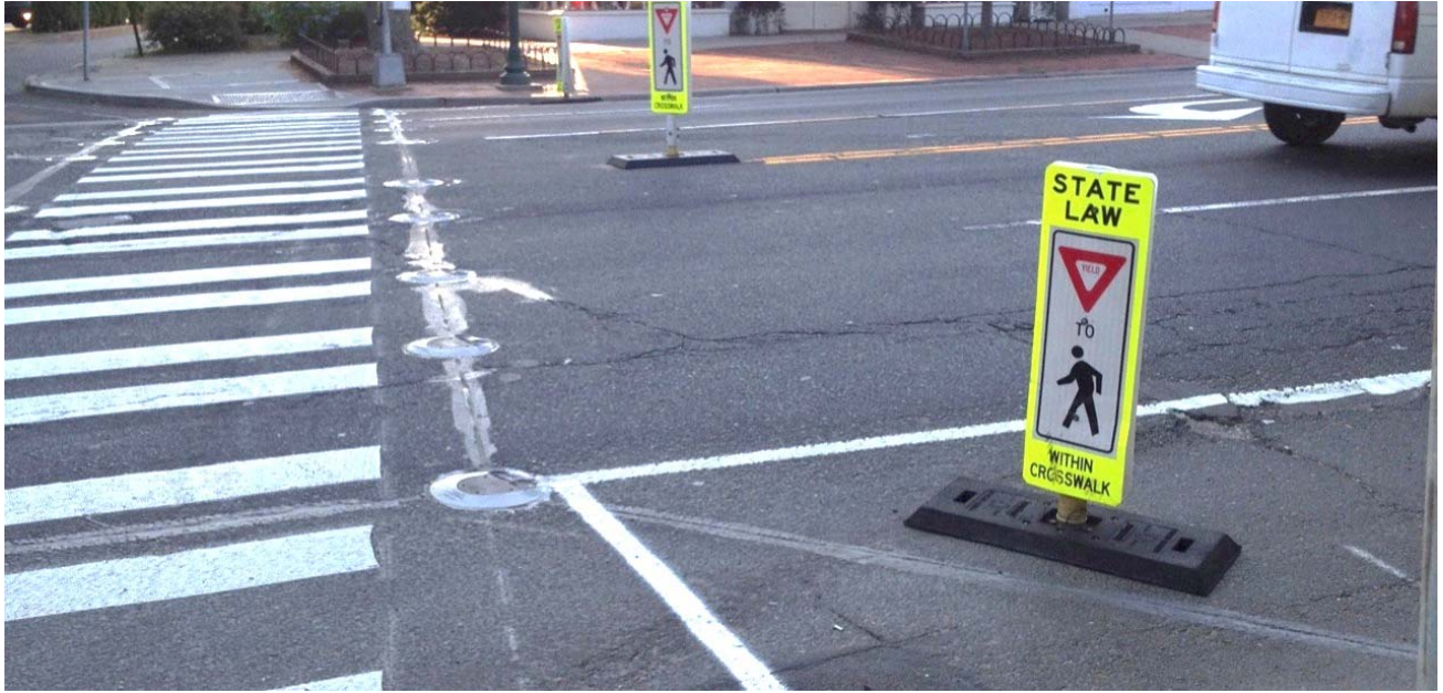
Figure 2. In-Roadway Warning Lights in the Village of East Hampton, NY
