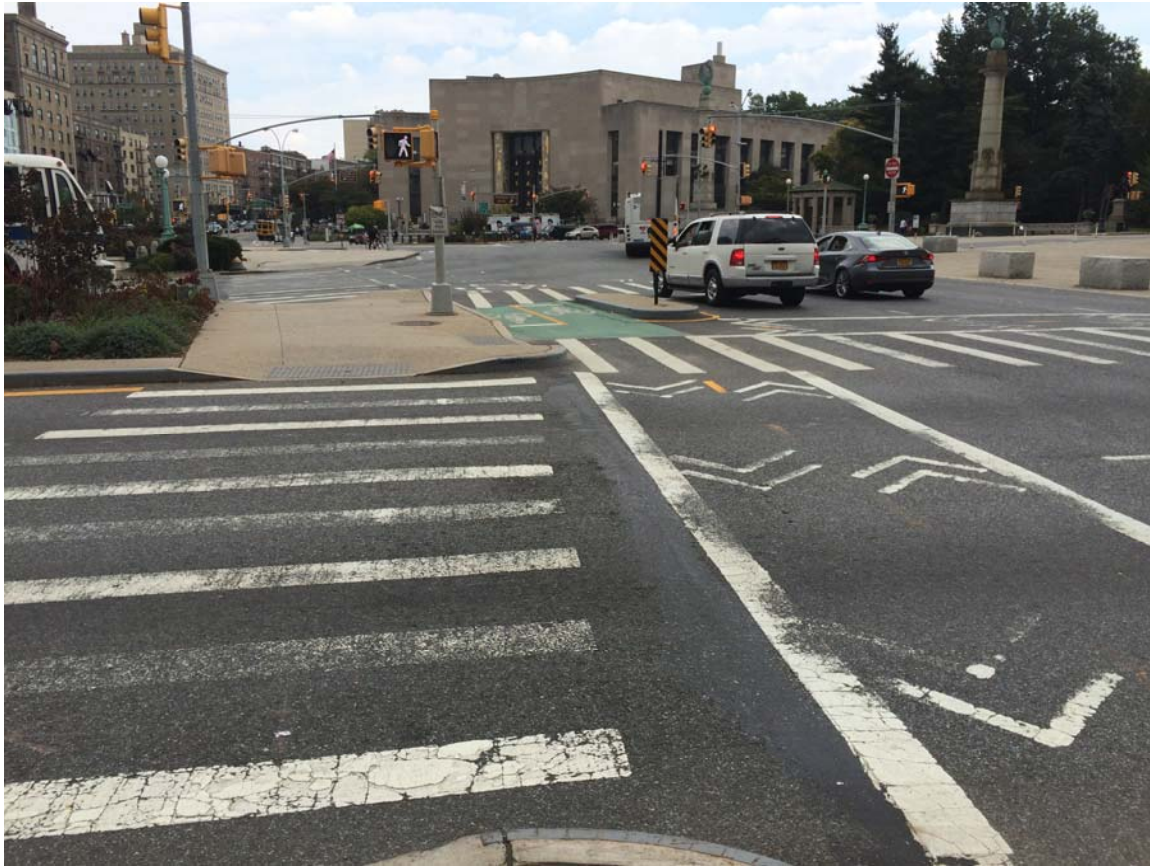
Figure 7. Crosswalk with adjacent bike lane (Grand Army Plaza, Brooklyn)
