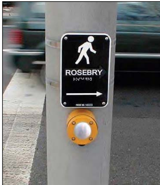
Figure 8. Braille street name legend above pushbutton [44].
