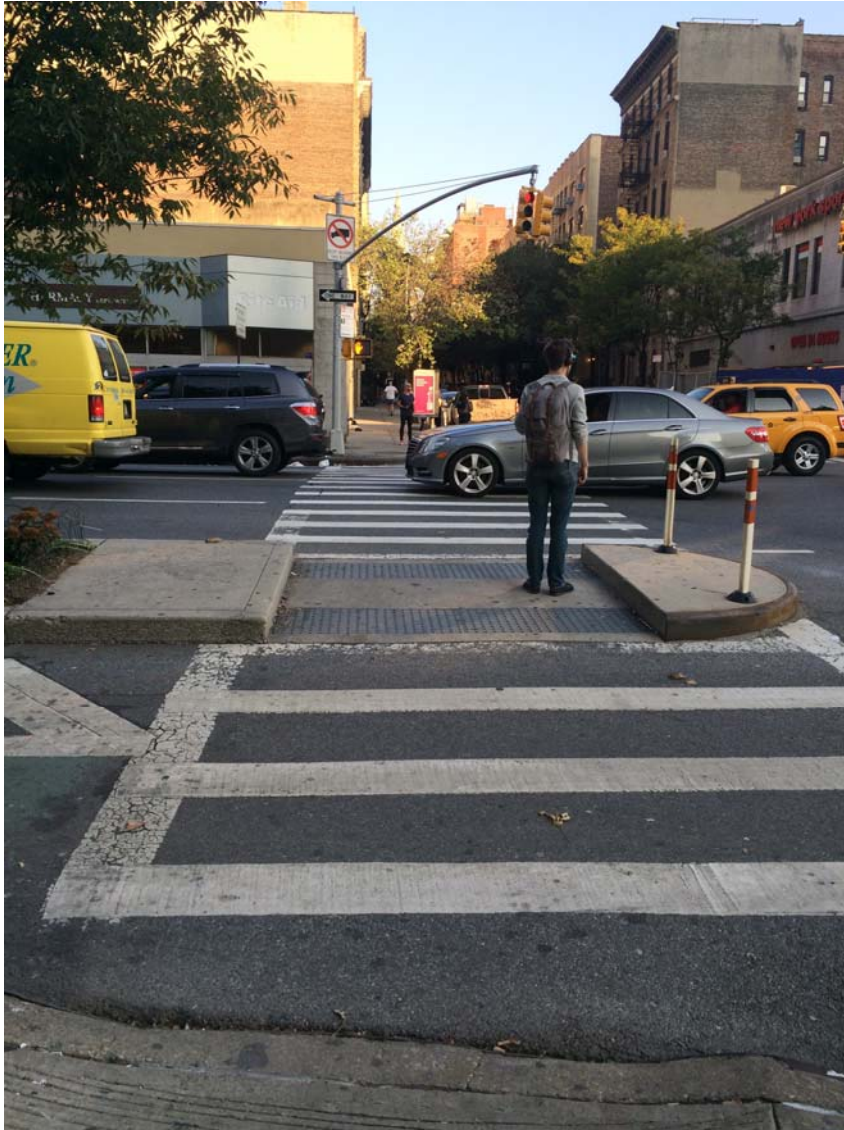
Figure 6. Pedestrian Island with bull nose located partially within crosswalk (Eighth Avenue at W.24 th Street, Manhattan)
