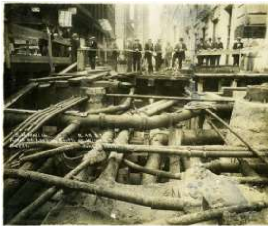
Figure 5. 1916/1917 Beekman Street Subway, NYC (Source: http://boingboing.net/2009/09/15/1917-beekman-street.html )
