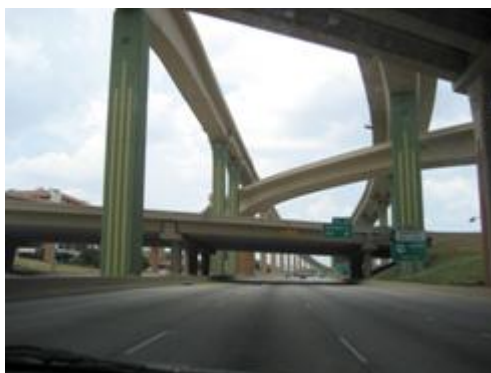
Figure 4.12: Full Control (Code '1'); all access via grade-separated interchanges
