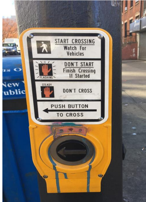
Figure 3.30 Accessible Pedestrian Signal (APS) Unit
