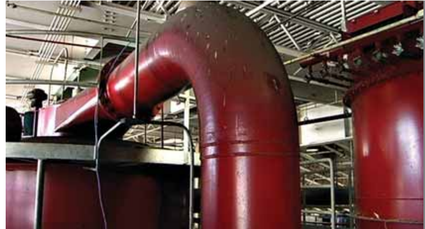
Photo by Greg Whitmore, 2010: Pneumatic Tubes Connecting to Cyclone Separators in Roosevelt Island Terminal
